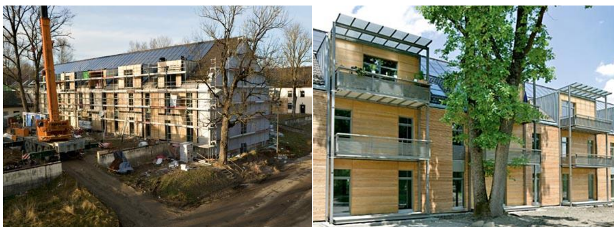
Fig. 5: Refurbishment of barracks buildings with prefabricated timber façade elements in Bad Aibling, Pictures: Huber & Sohn 161
