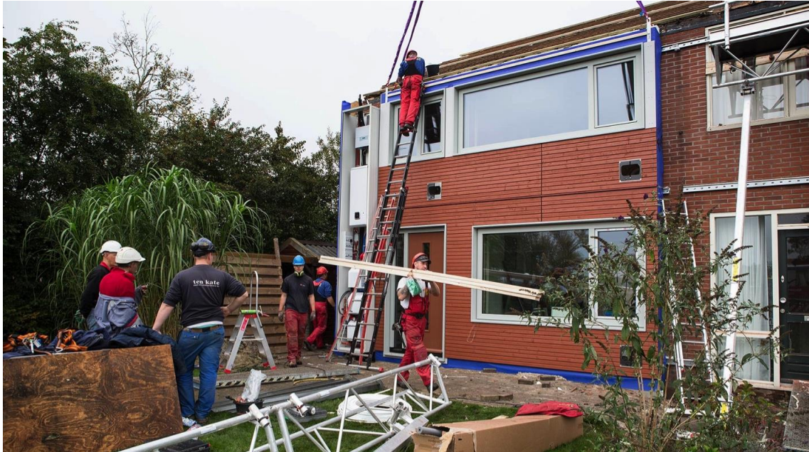
Mounting façade elements on a building in Nieuw Buinen and the Smart Portal (left) including the heating and ventilation equipment, © Photo: Frank Hanswijk, Source: Flickr 156
